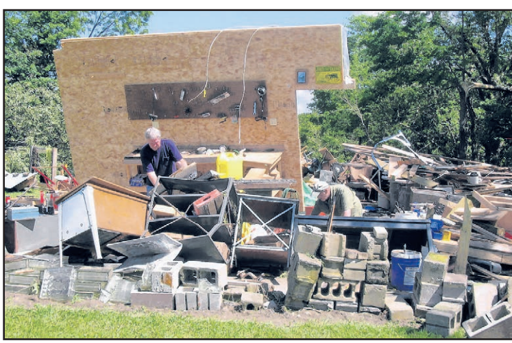
Mitch Hessinger surveys the damage of his leveled garage on Michigan 62 between Cassopolis and Dowagiac Monday. Hessinger was working in his garage Saturday night when a tornado tore the garage down. Hessinger was standing in the doorway, pictured at left, when the garage collapsed.
