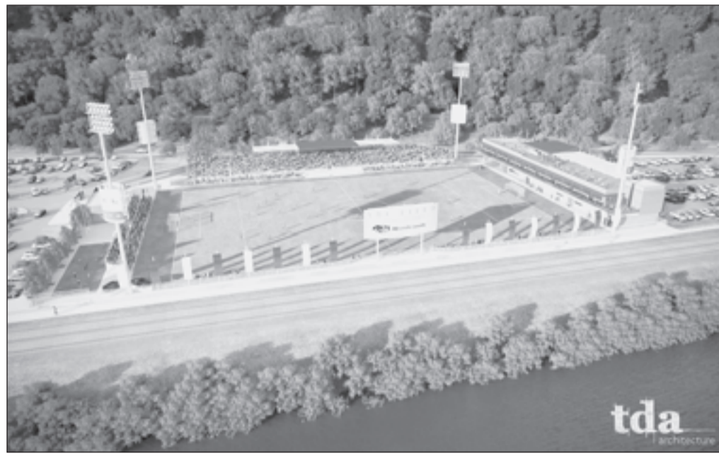
A view of the future Highmark Stadium in Station Square. The stadium should be ready for play sometime this fall.
